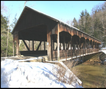
Covered Bridge over Clear Fork Gorge River
